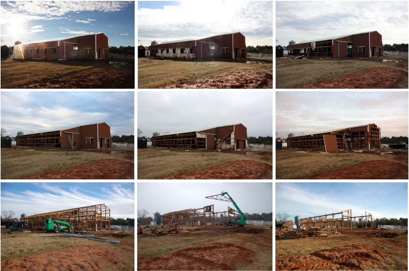
Figure 5: Selected time-lapse photos illustrating different stages in the deconstruction sequence: View from the north
